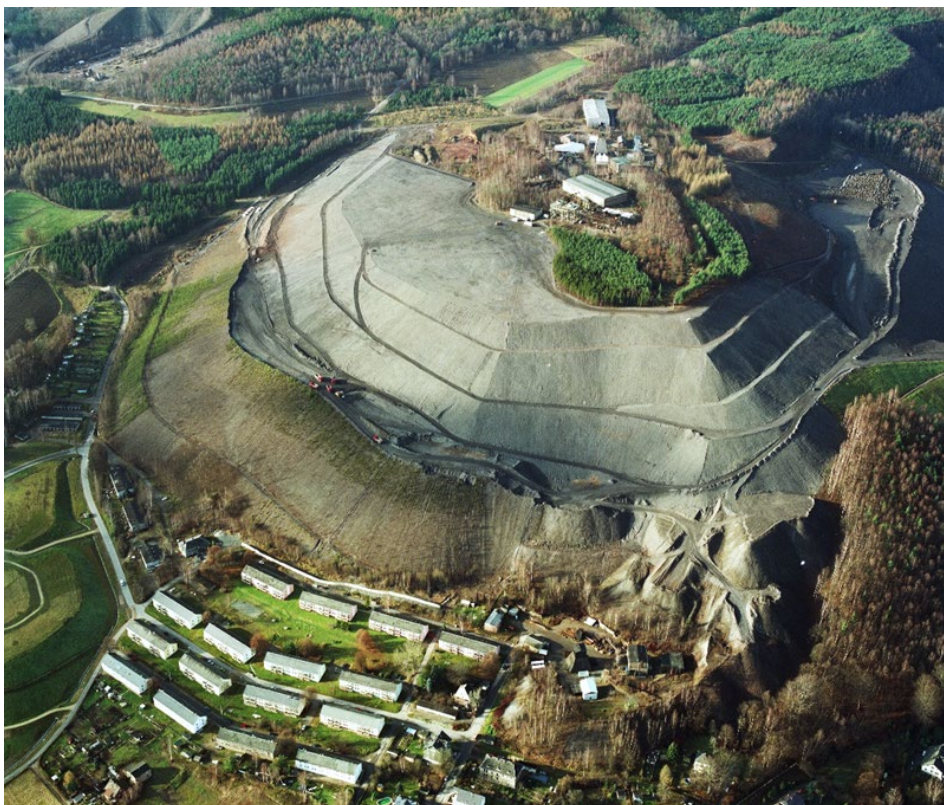
FIG. I-2 Waste rock pile and shaft n° 382 in 2000, three years after start of remediation activities (contouring) (Archive Wismut GmbH).
