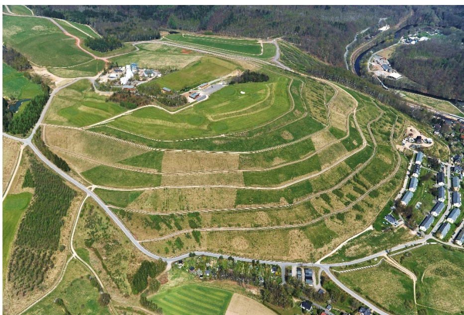
FIG. I-5 Waste rock pile and shaft n° 382 in 2010, showing covering works completed and the revegetation step (Archive Wismut GmbH).
