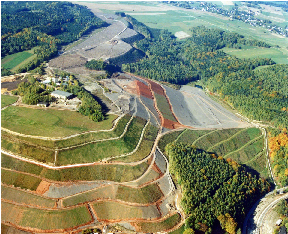
FIG. I-3 Waste rock pile and shaft n° 382 in 2003, showing contouring works and installation of the cover ( Archive Wismut GmbH ).
